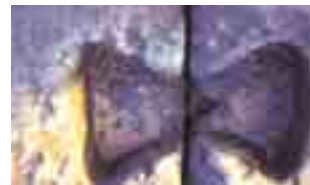
Imprint of metal clamp on stone structures at Angkor Wat, Cambodia
